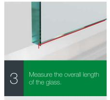
Check this measurement in a few different places, as the gap can sometimes vary in size.
